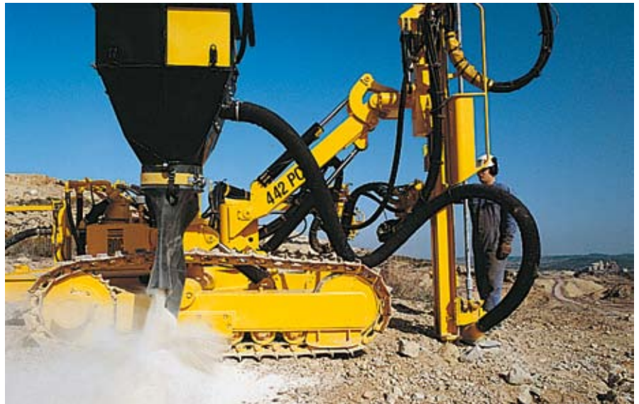
Dust collector for better working environment
